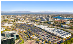
3. Bridgepointe Shopping Center San Mateo, CA
